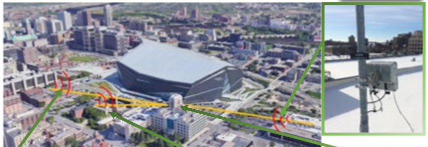
Remote rooftop site
