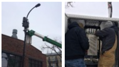
Small cell on light pole
